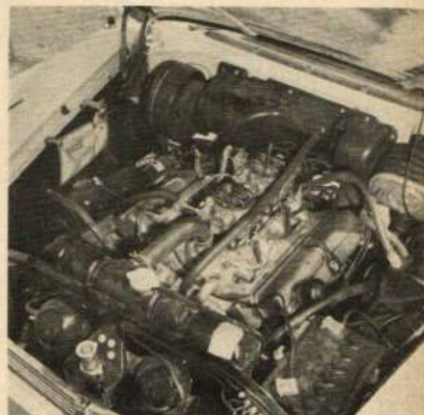
318-cubic inch Fury engine with two four-barrel Carters. Two dry-mesh air cleaners are used here and are practically silent.
