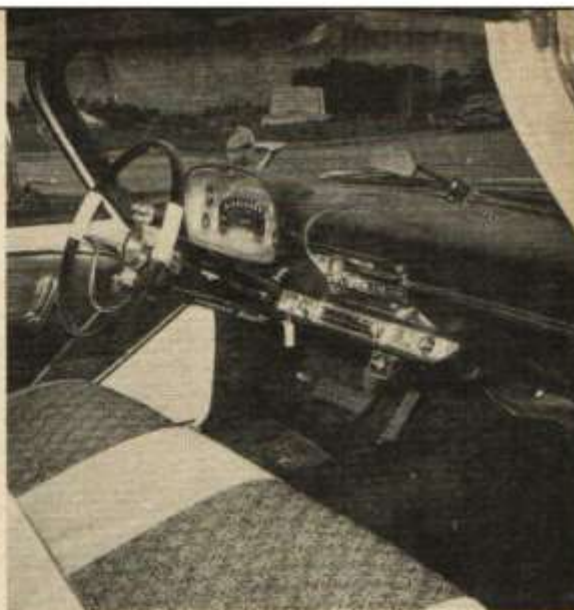
Interior layout of standard Plymouth cab. Ease of access, fairly good comfort, excellent forward visibility were noticed.
